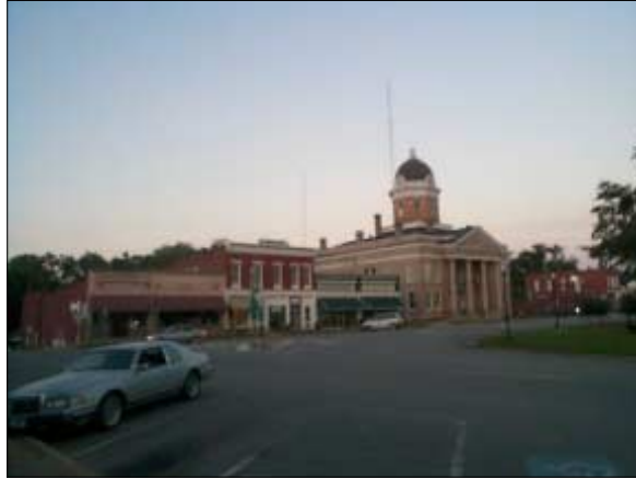
North side of Green Street flanking the central square features a range of commercial buildings, including the high-style Jasper County Courthouse. Note that brick construction and storefronts at street level are the predominant visual characteristics.
